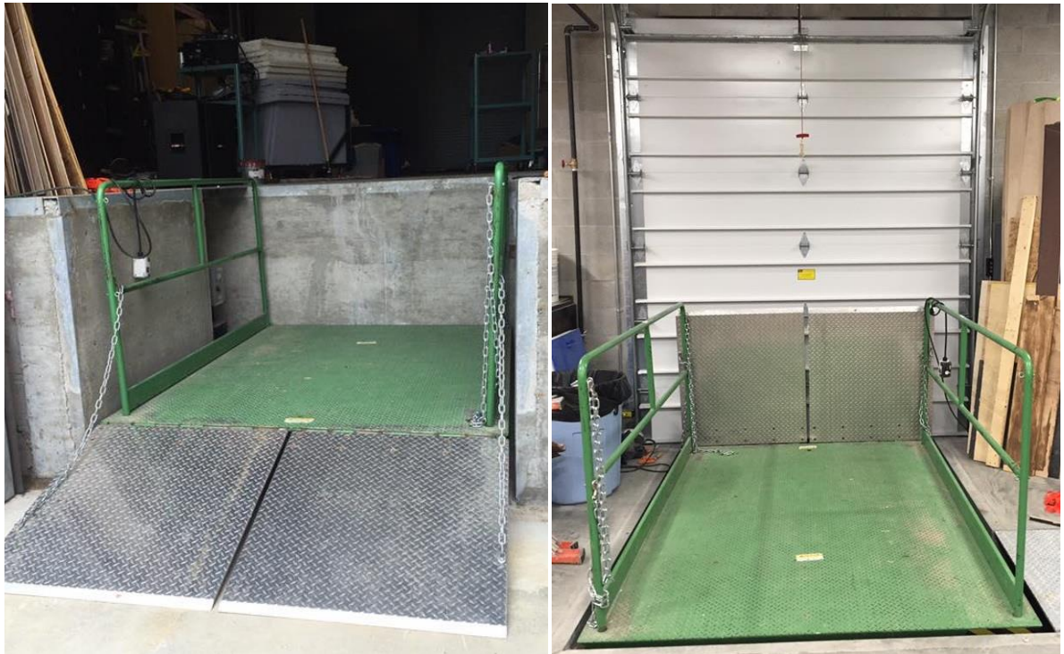
Lift lowered for ground level load-in. Railings are removable.
