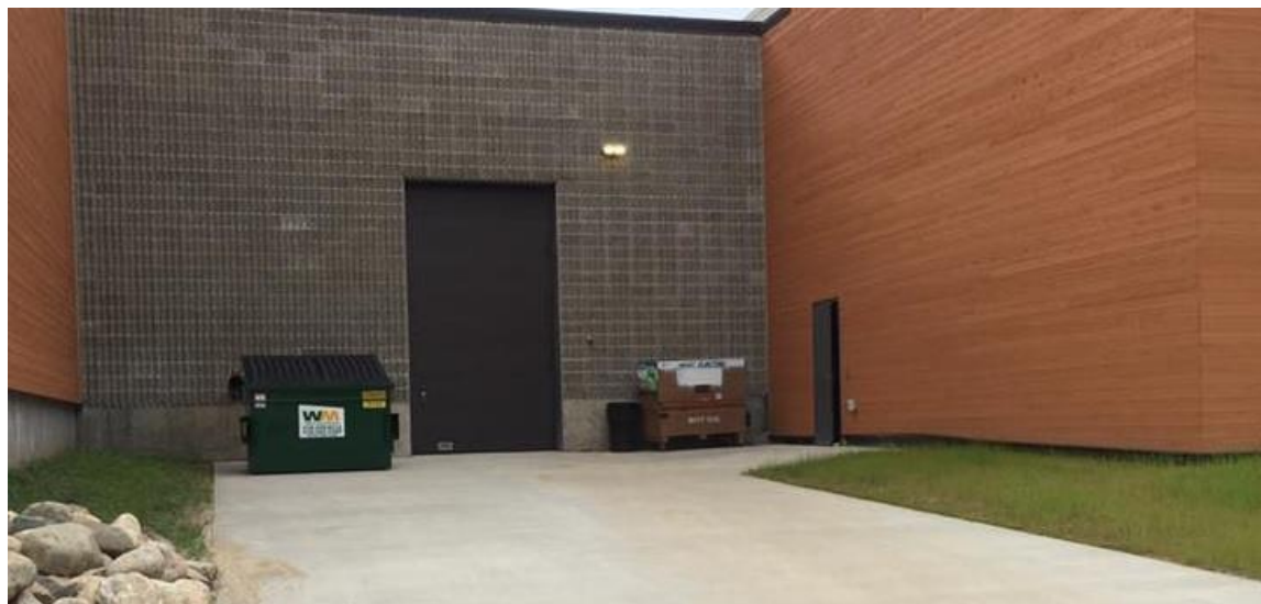
Loading Dock and approach
