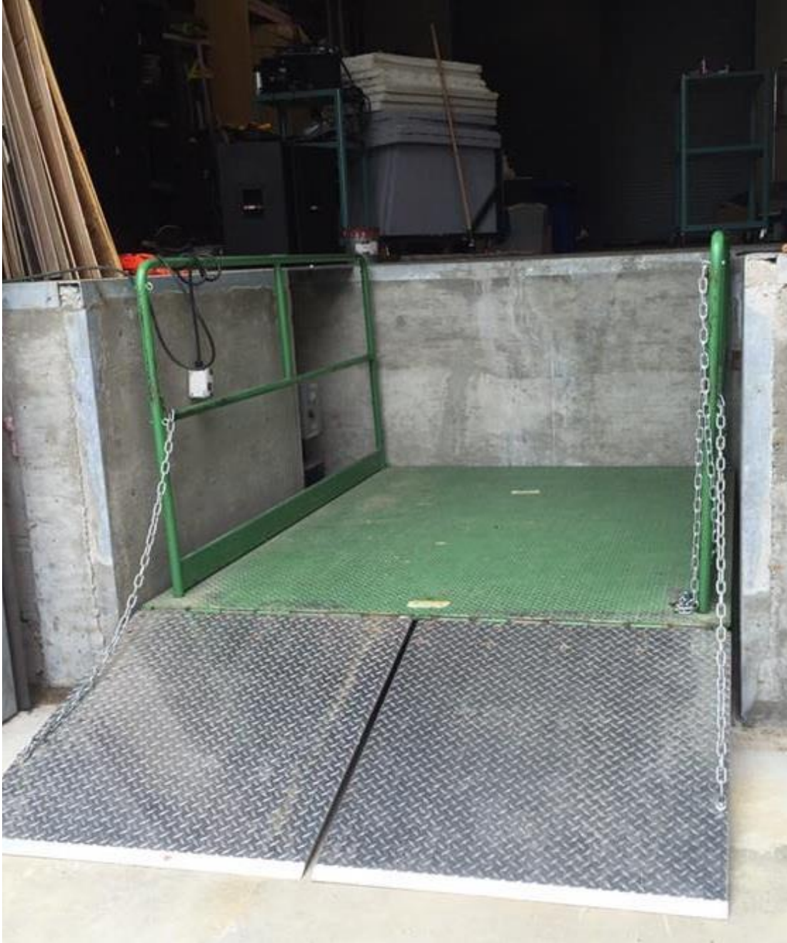
Lift lowered for ground level load-in. Railings are removable.
