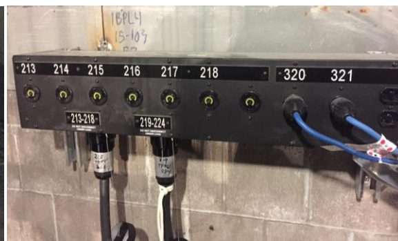
Pin Rail Multipin/Twistlock Circuits and Relay Circuits
