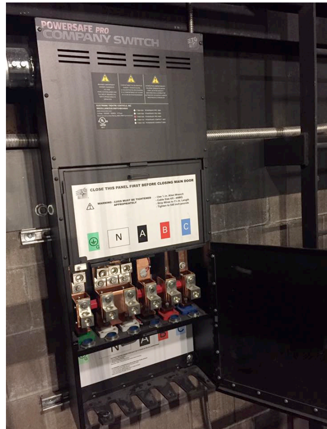
400 Amp Company Switch on Pin Rail
